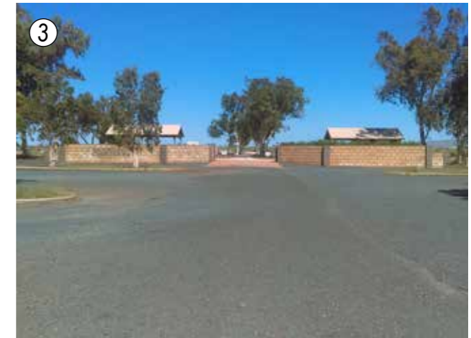
3 View of entrance from carpark
