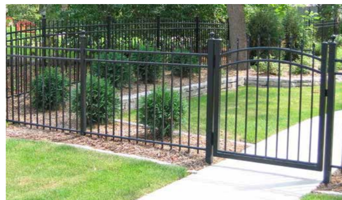
Steel boundary fence with pedestrian gate
