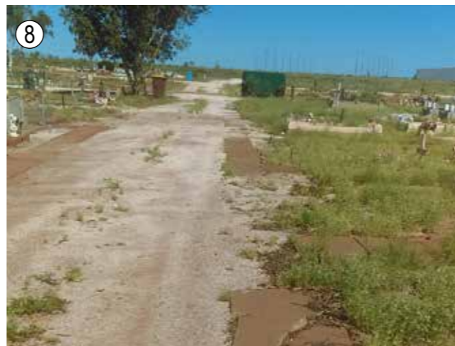
8 Western internal road and pathway
