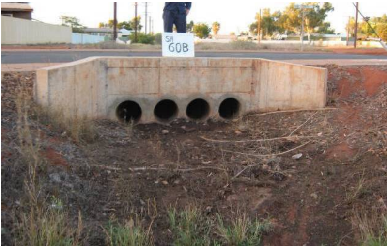
Plate 10 – SH60 under Brodie Crescent
