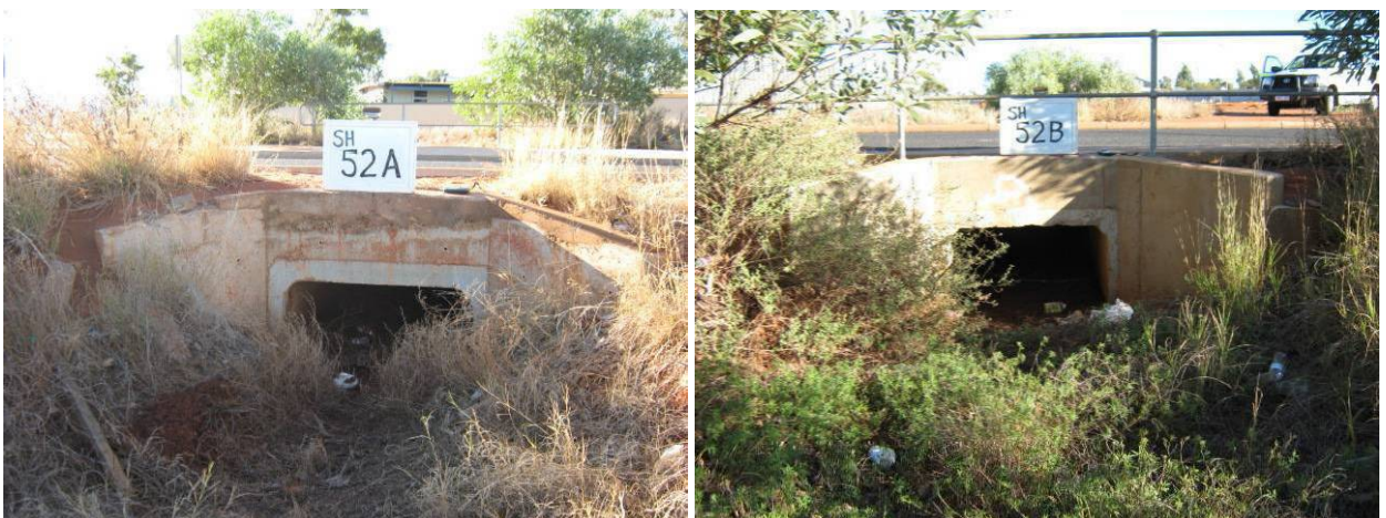
Plate 11 – SH52 under Brodie Crescent
