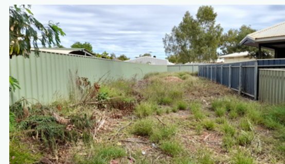
Western facing view from mid portion of PAW
