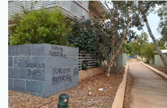
Southern facing view from Smith Street
