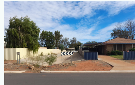
North westerly facing view from Paton Road
