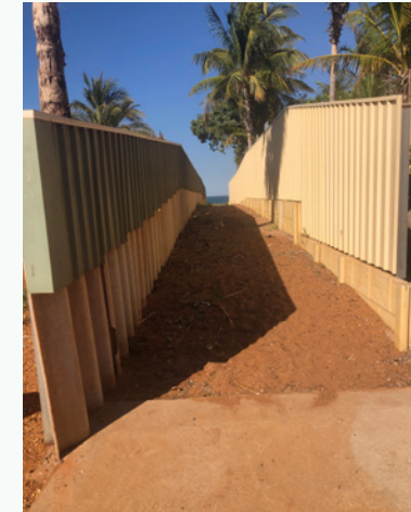
Rawlings Close frontage
