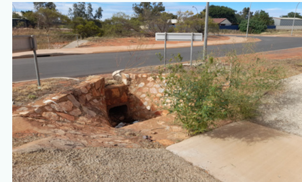
Drainage on Paton Road
