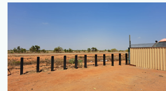
Ashburton Court frontage to northern portion of PAW
