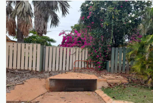
View from Brodie Crescent
