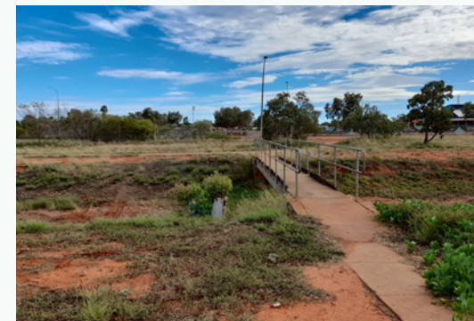
Pedestrian bridge north of PAW on drainage reserve
