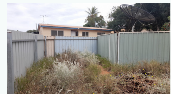
South eastern view from western lot
