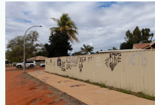
Southern facing view of southern portion of PAW (Northern Land)
