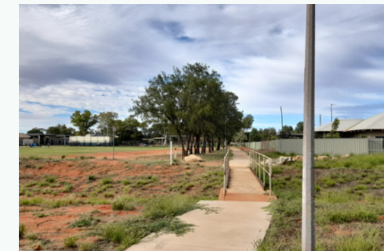
Pedestrian bridge over drainage reserve to the south of PAW to access Baler Primary School
