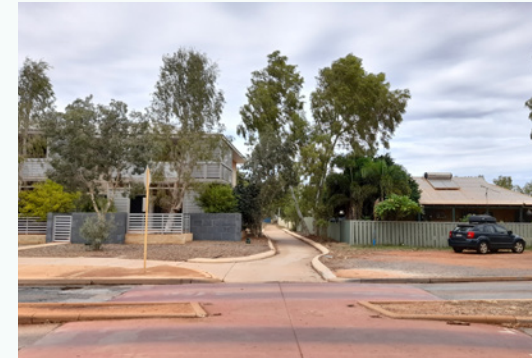
Southern facing view from Smith Street
