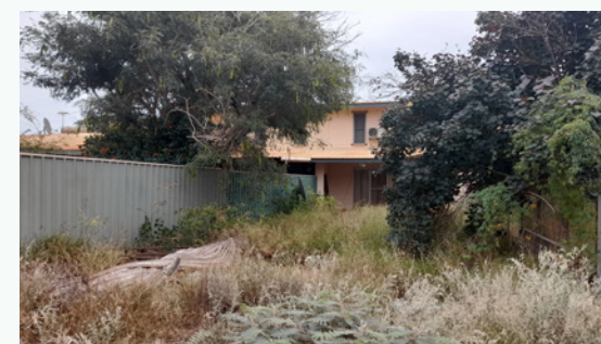
Northern view from western lot
