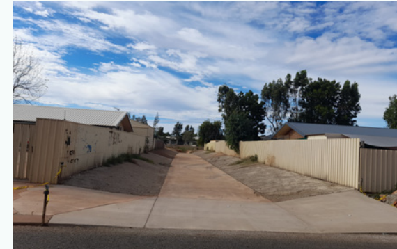
South easterly facing view from Limpet Crescent
