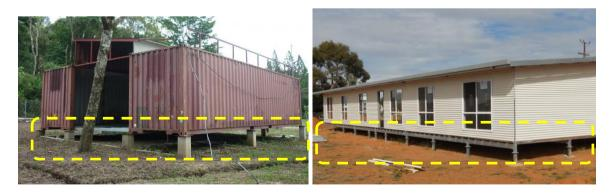
Not permitted in Scenario B, C, D, G, H & I – exposed subfloor void for shipping/sea container and other transportable building
