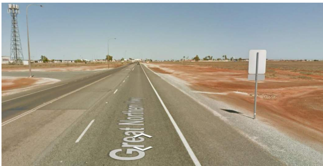
Figure 21 Existing Great Northern Highway – view of the westbound approach to the Highway Precinct Access Road intersection (source: Google Streetview)
