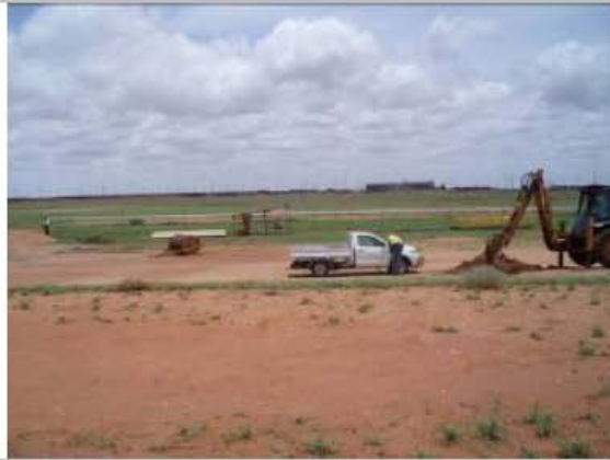
Photo 1: Test pit 1 at MSSR. View facing East.
