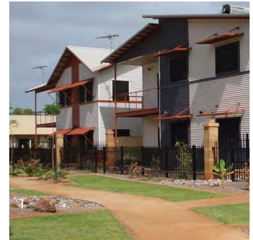
Passive Surveillance of Pedestrian Access Way
