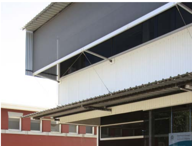
A combination of shading devices are used to shade both glazing and walls.
