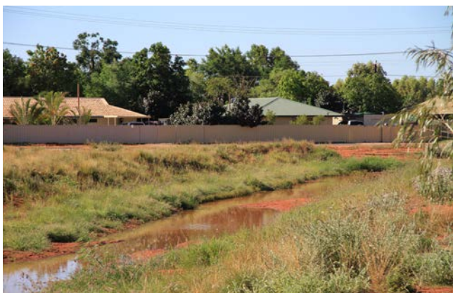
South Hedland drainage swale after rain.
