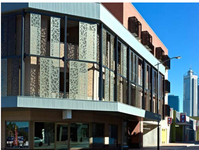
Foundation Housing artwork by CODA + Olga Cironis integrated into the building form.
