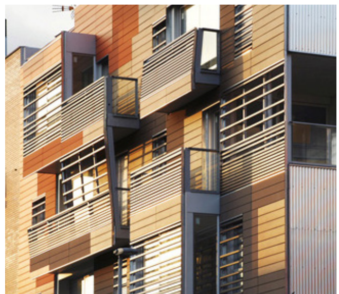
An example of insulated lightweight construction with a range of balcony types that also break up the long facade and provides interest with a mix of materials and colours.
