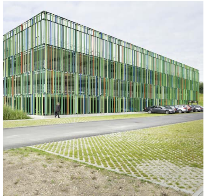
An example of screening on a decked carpark structure, Germany.
