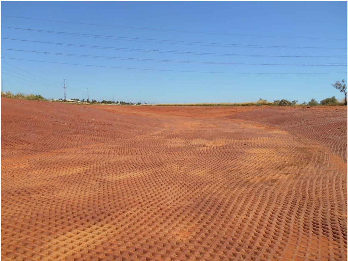
Figure 3-3 Constructed Drainage Channel
