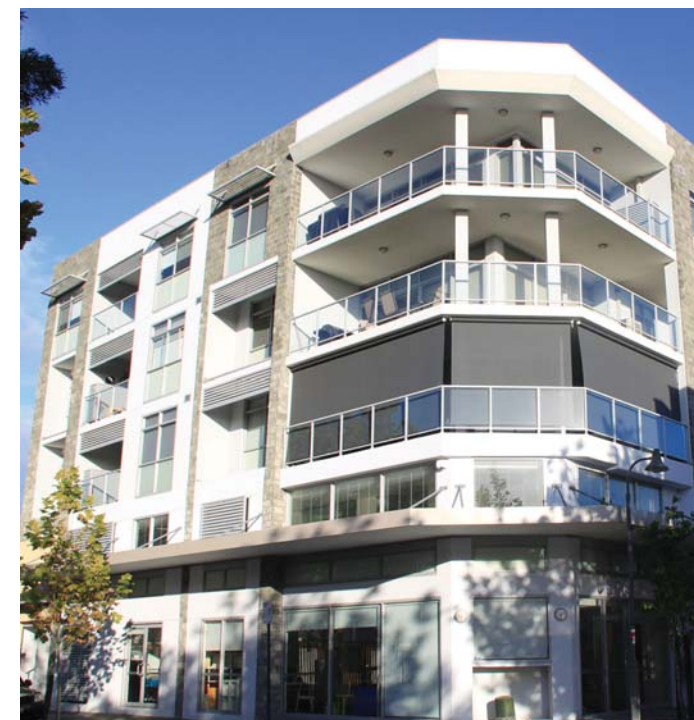
Figure 36: Example of Mixed Use Development
