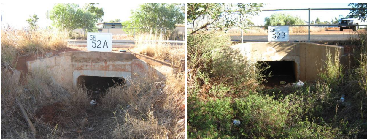
Plate 11 – SH52 under Brodie Crescent
