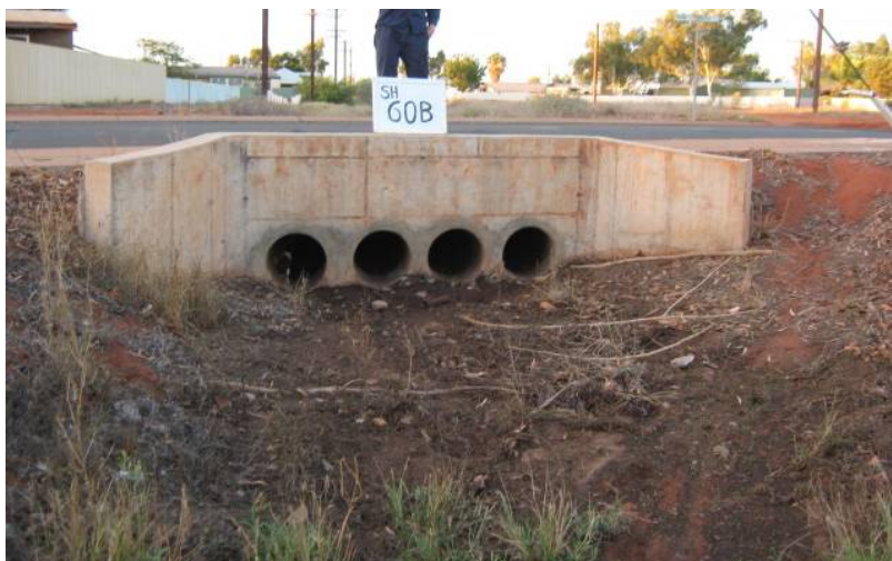
Plate 10 – SH60 under Brodie Crescent
