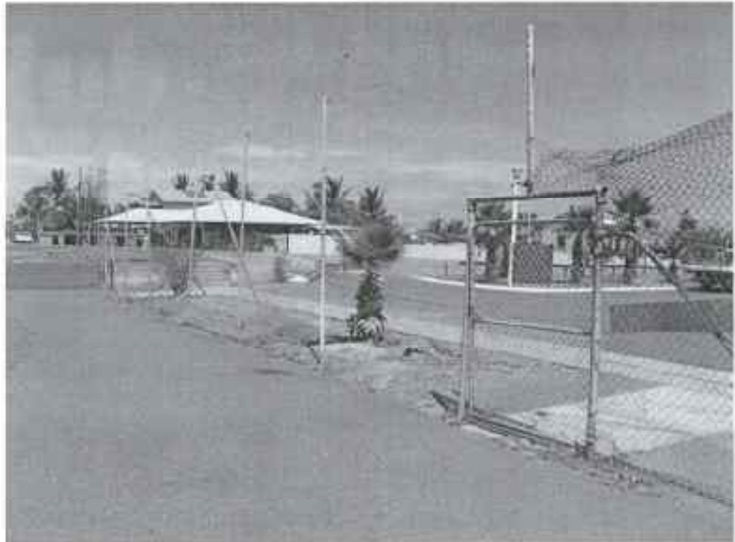
Further damage to tennis court fencing and fence poles
