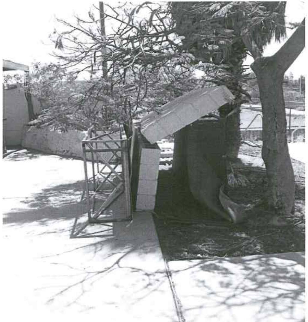
Concrete block wall blown over during Cyclone George
