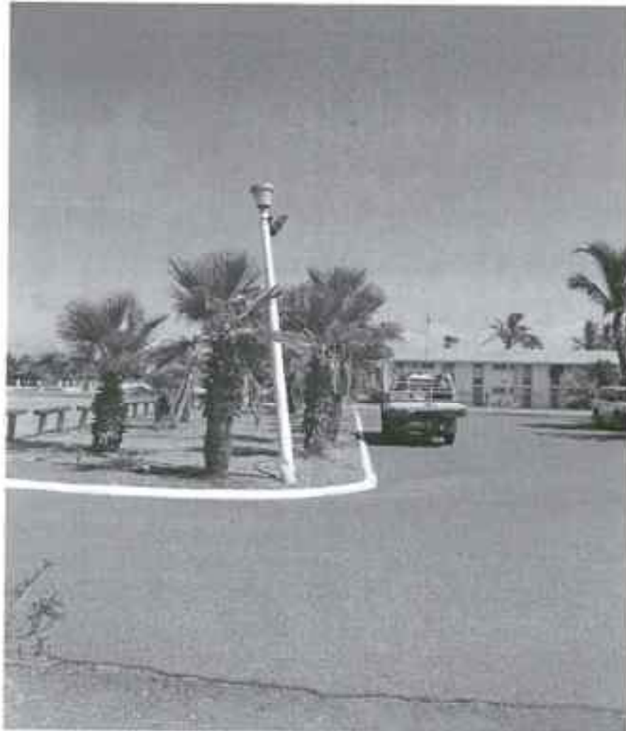
The above pole was bent during Cyclone George
