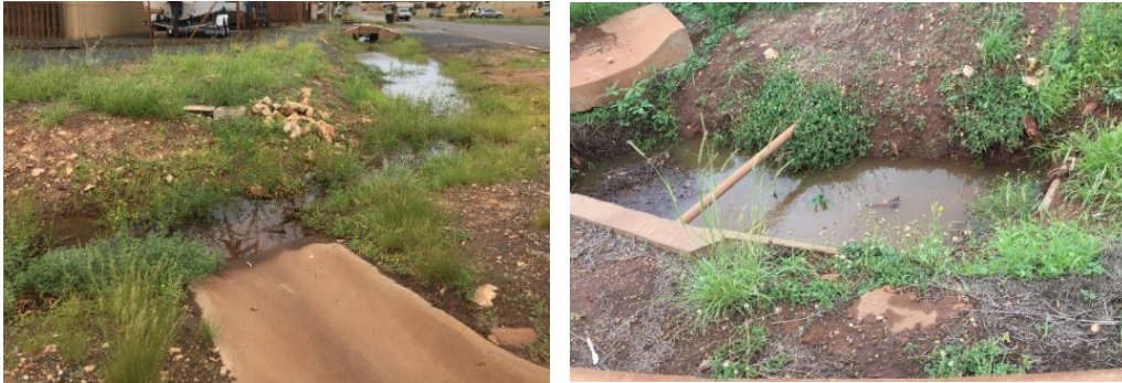
Figures 9 & 10. Stormwater drains at Wilson St Port Hedland.
