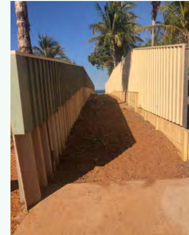
Rawlings Close frontage
