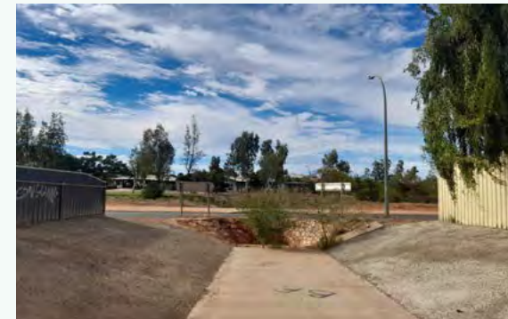
South easterly facing view over Paton Road
