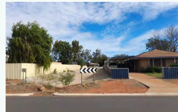
North westerly facing view from Paton Road
