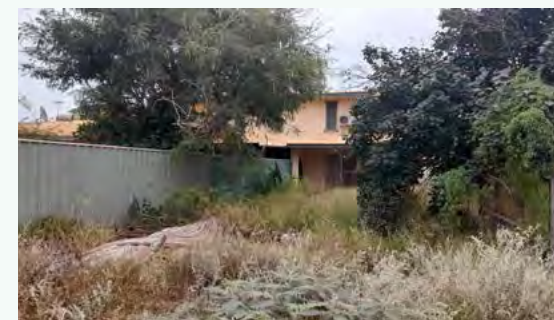
Northern view from western lot
