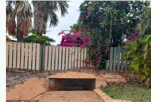
View from Brodie Crescent
