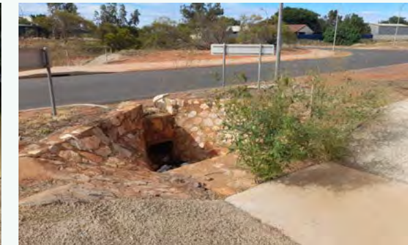
Drainage on Paton Road
