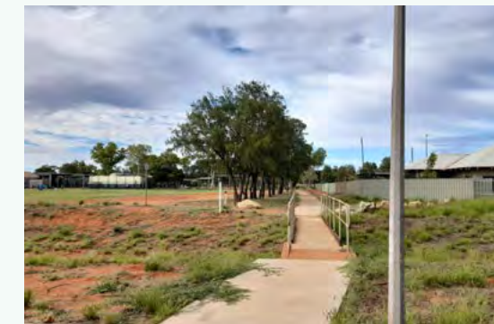
Pedestrian bridge over drainage reserve to the south of PAW to access Baler Primary School
