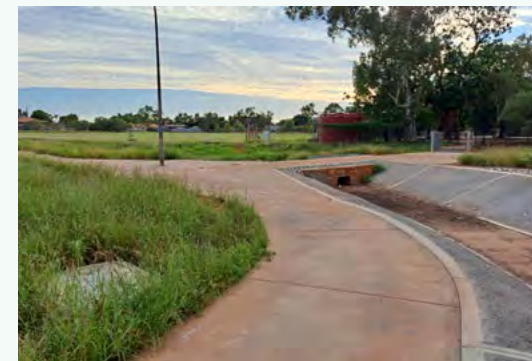
North eastern facing view from mid section of PAW
