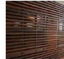
T2- TIMBER BATTEN SCREEN - STAINED FINISH
