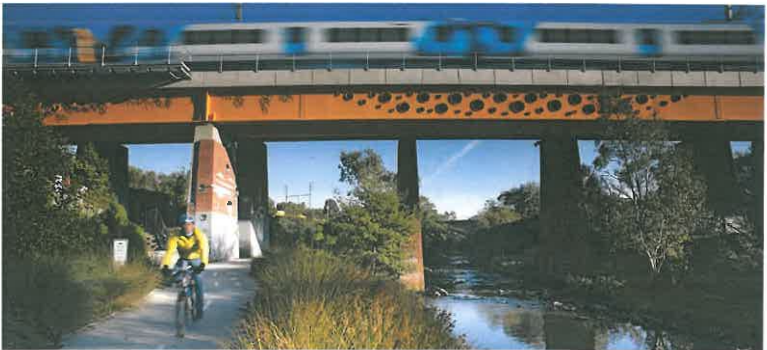
Clifton Hill Rail Duplication Project Winner: AILA Vic. Urban Design Award 2011, AILA National Design Award 2012 BPN (Building Product News) Sustainability Awards, Landscape Design Award 2012
