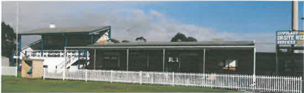
Existing conditions - before demolition
