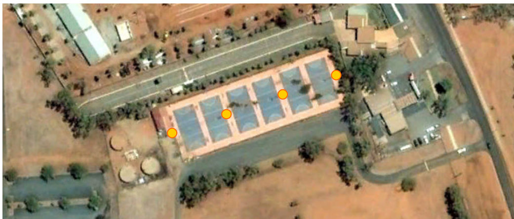
Figure 10: Faye Gladstone Netball Courts
