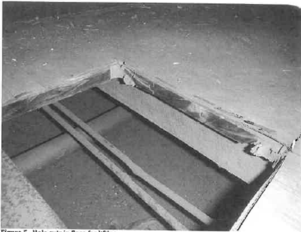
Figure 5 - Hole cuts in floor for lifting
