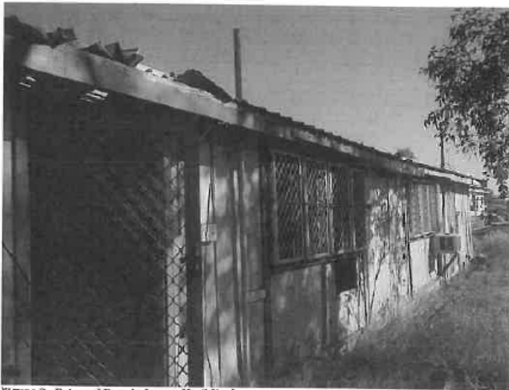
Figure 3 - External Facade (rear of building)
