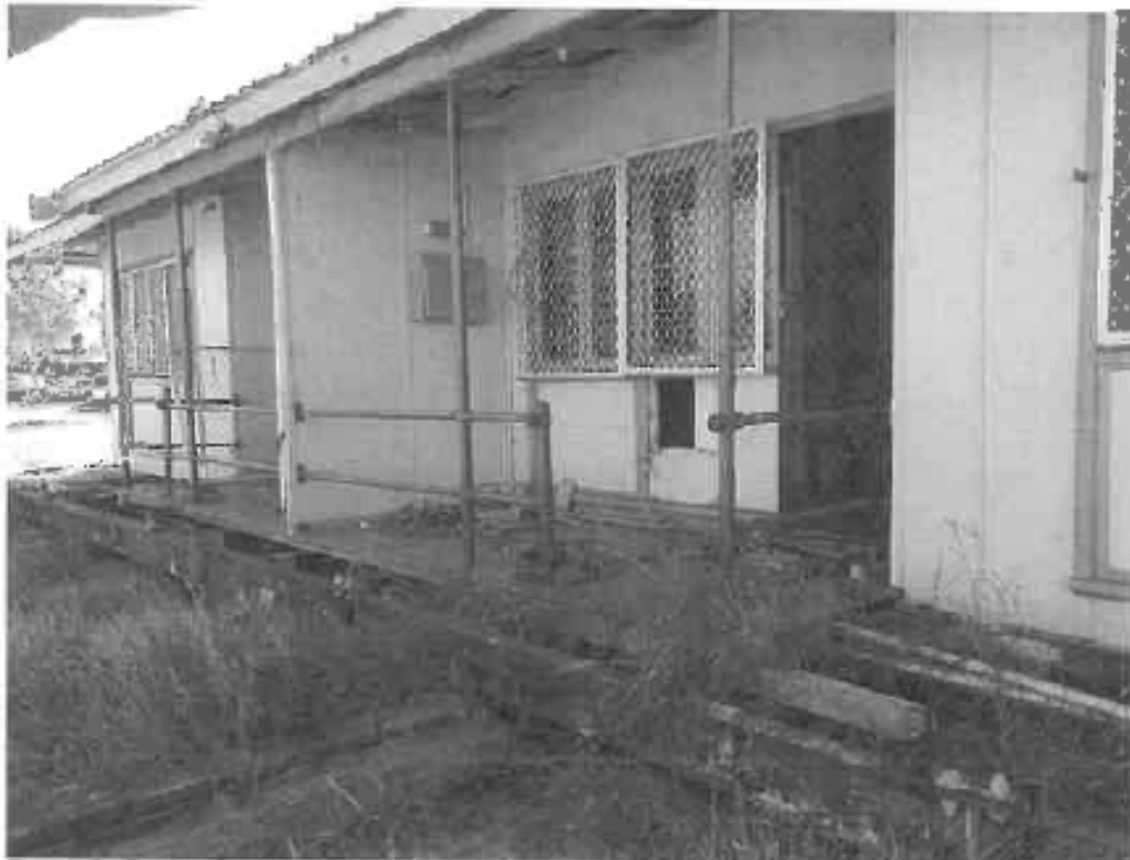
Figure 2 - External Entry and Verandah
