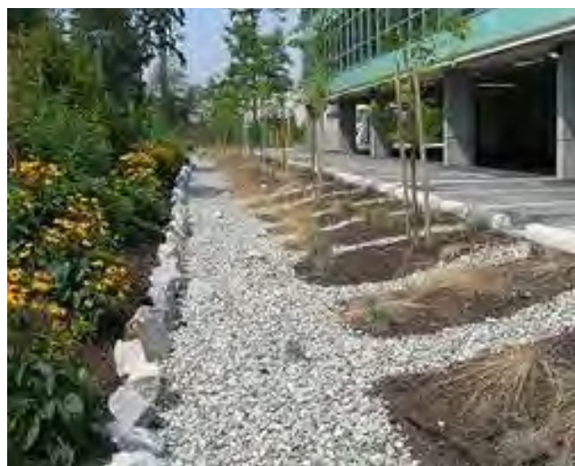
An example of stormwater detention within a lot. Appropriate design to address the heavy deluges of rain during the cyclone season is required.
