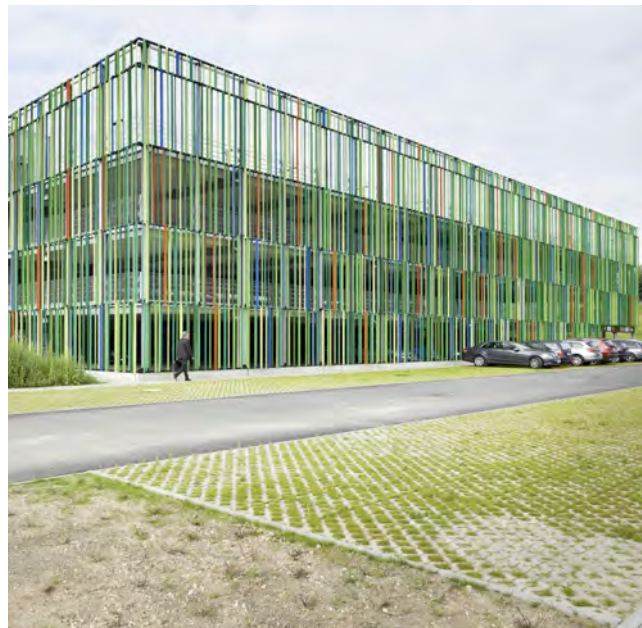
An example of screening on a decked carpark structure, Germany.
