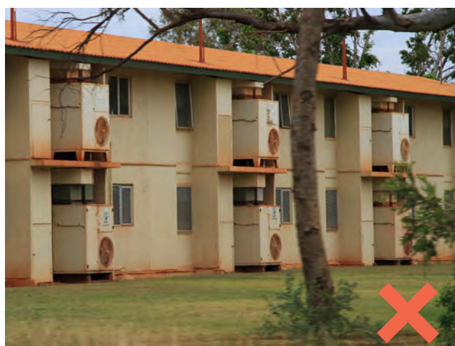
Air conditioning condenser units must not be viewed from the street in the Town Centre.
