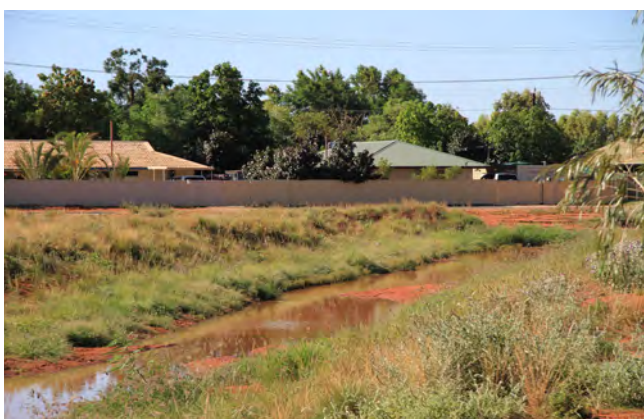
South Hedland drainage swale after rain.
