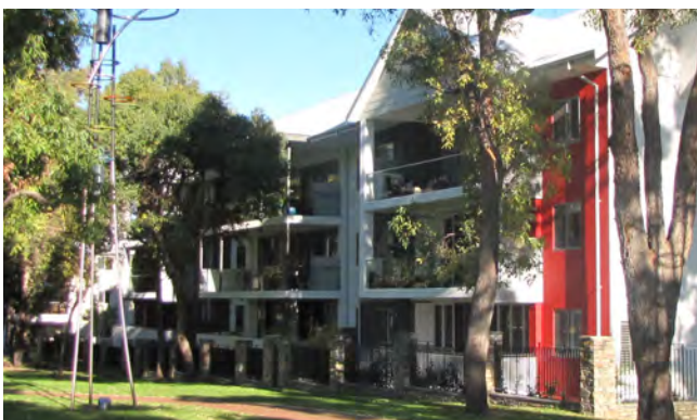
Opportunities for effective public realm surveillance by locating balconies adjacent to POS.
