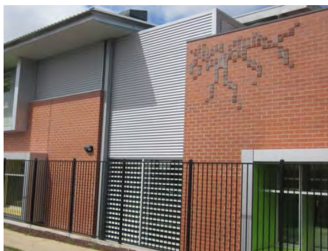
Examples of service enclosures and screening treatments designed as an integral part of the overall development.
