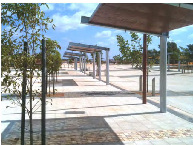
Trees and shade structures will assist in minimising reflected heat load. Choose Seating, bollards, rubbish bins and paving for open spaces that are robust and complements the South Hedland Town Centre public environment - Wise Terrace, South Hedland.
