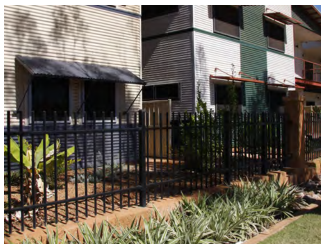
Permeable fencing provides passive surveillance opportunities for this group dwelling development in Port Hedland.
