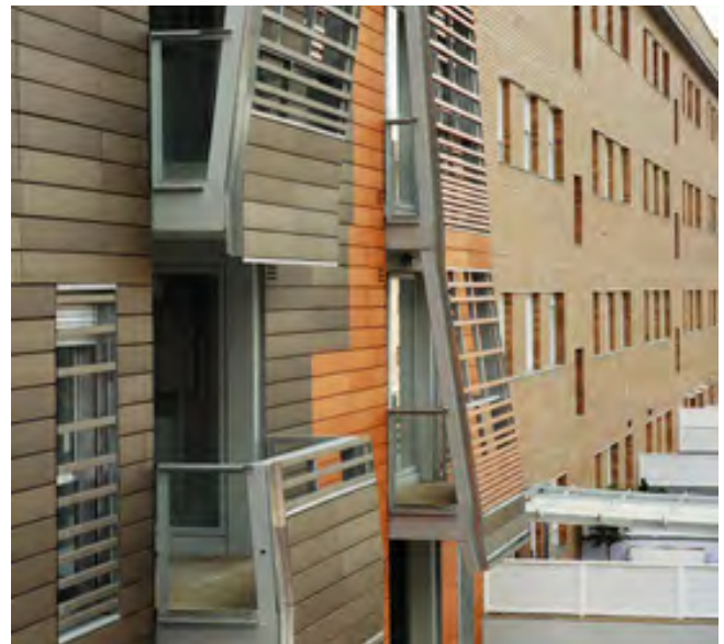
An example of building elements (balconies) integrated into the overall building form and adds interest to a long plain facade.
