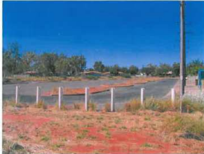
Picture 1. Catamore Court road reserve and carpark
