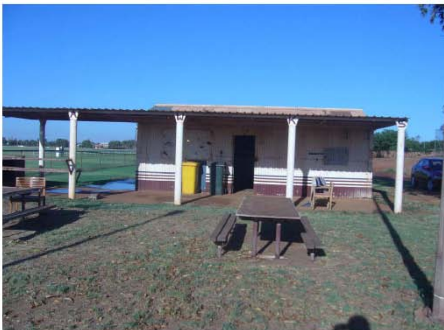
Photograph 2 East Elevation McGregor Street Shed, Port Hedland Carrick + Wills Architects February 2010
