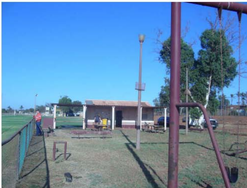
Photograph 6 East Elevation with playground in foreground McGregor Street Shed, Port Hedland Carrick + Wills Architects February 2010
