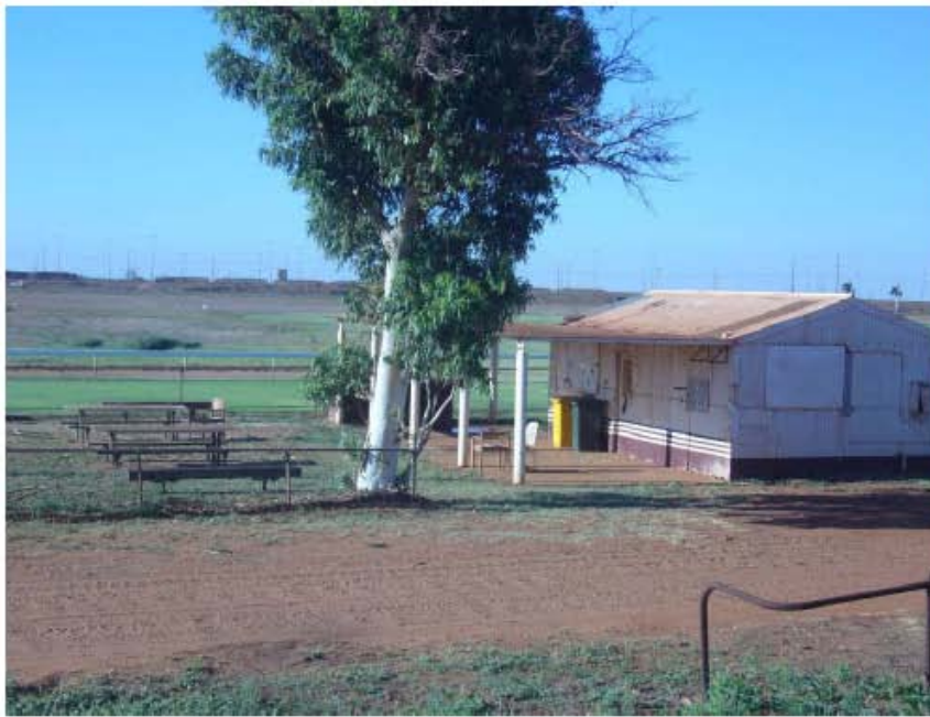
Photograph 7 North-East Elevation McGregor Street Shed, Port Hedland Carrick + Wills Architects February 2010
