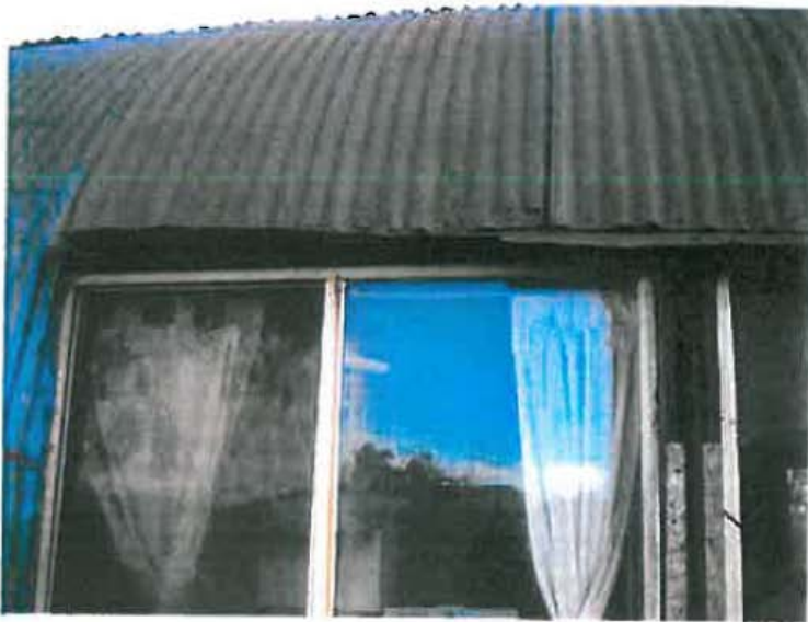
Front detail showing aluminium framed windows.
