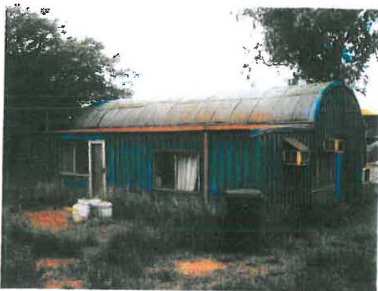
View looking to southeast showing rear extension along the north.
