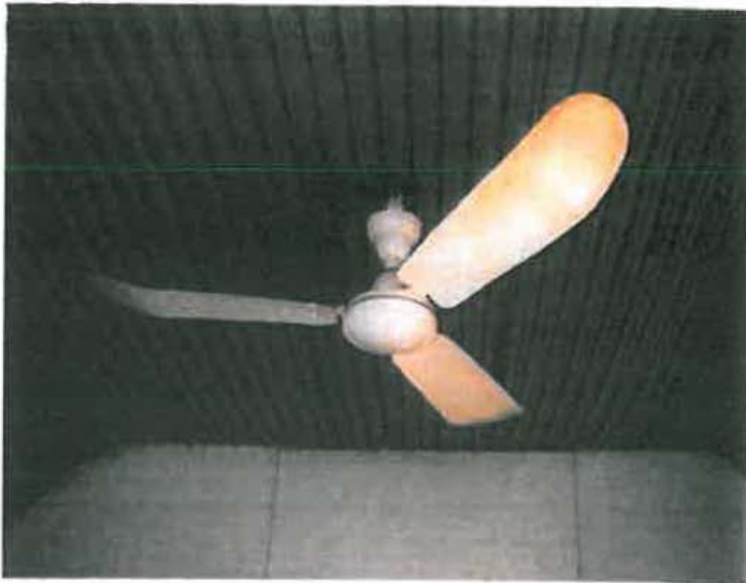
Interior: Covered ceiling lining in Nissen hut.
