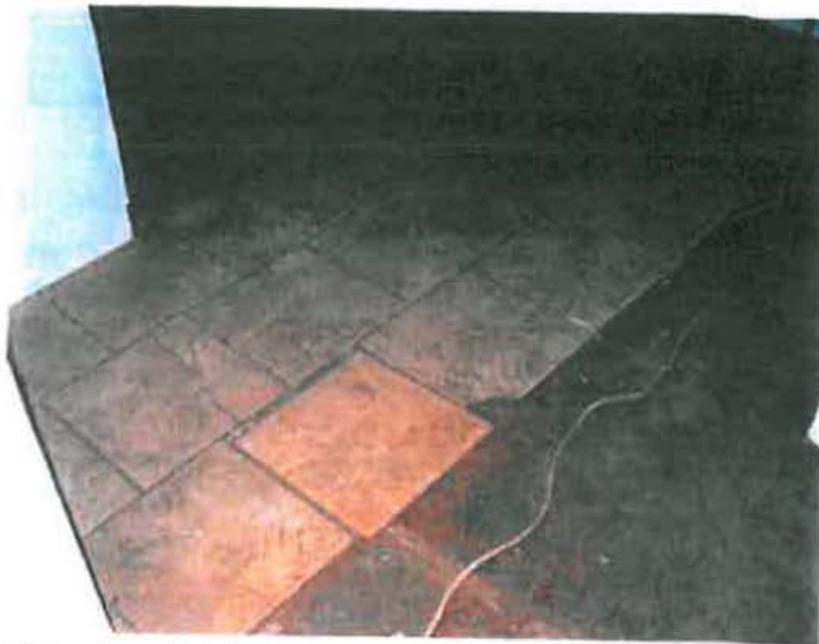
Interior: floor detail showing bare concrete and ceramic tiles.
