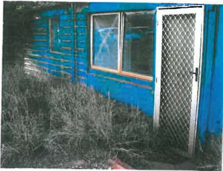
Detail of northeast corner of the extension
